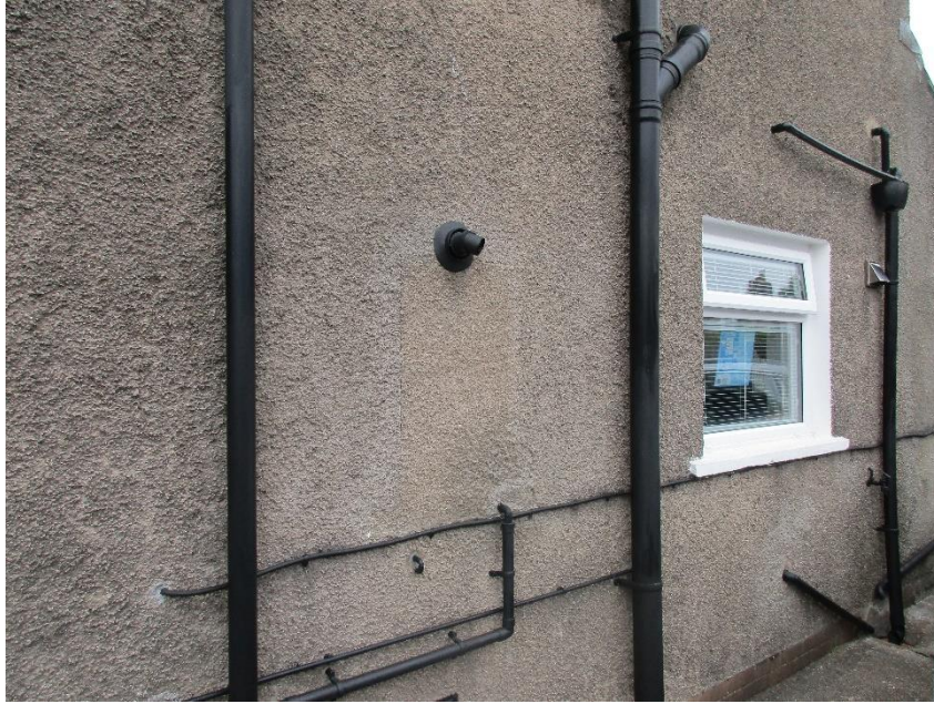
21 Exterior – Evidence of window infill to side elevation.
