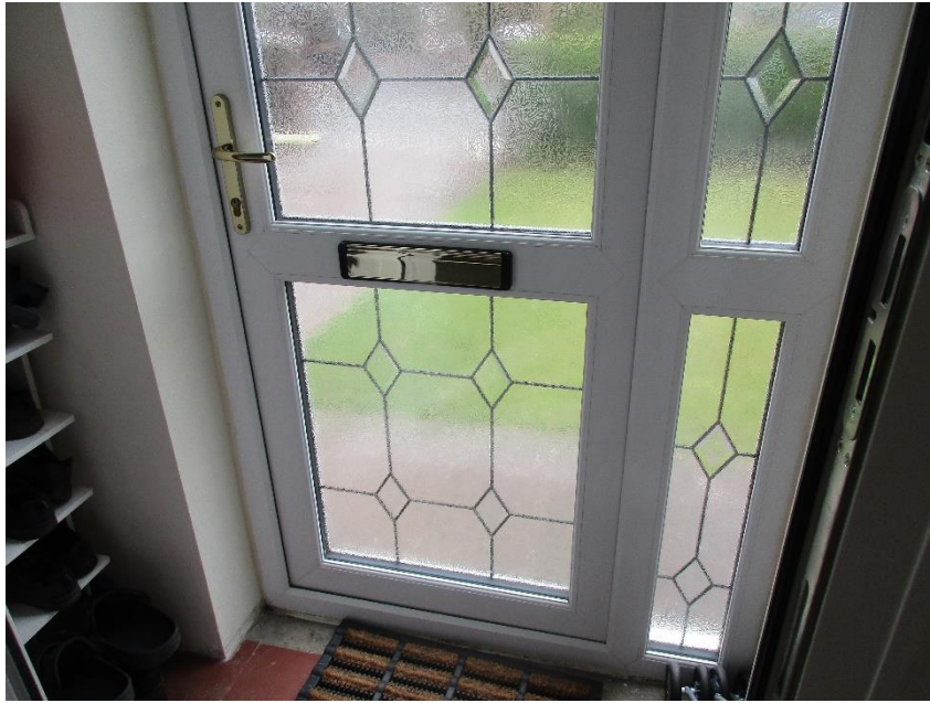
51 Interior – Entrance Porch.
