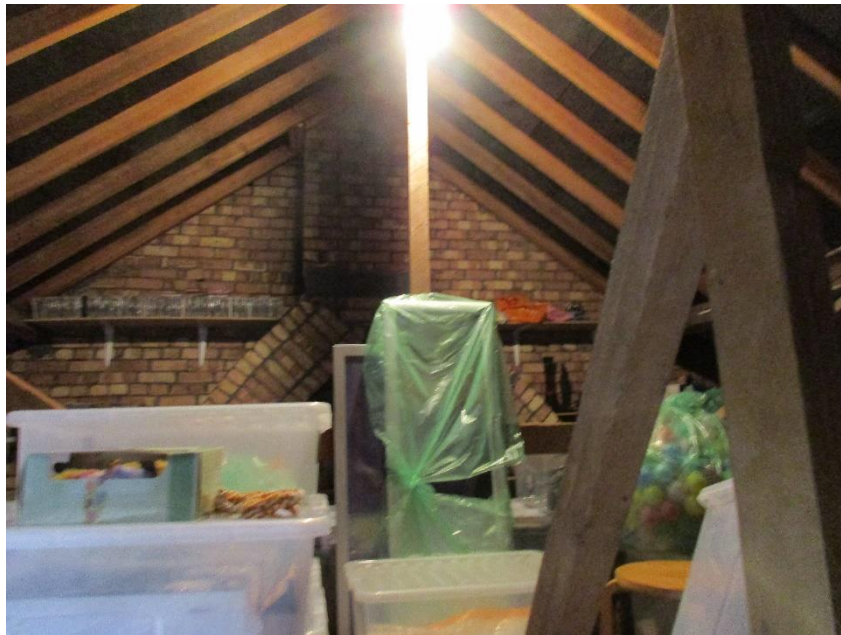
10 Interior – Roof Void – Cut timber roof structure and bituminous under felting.
