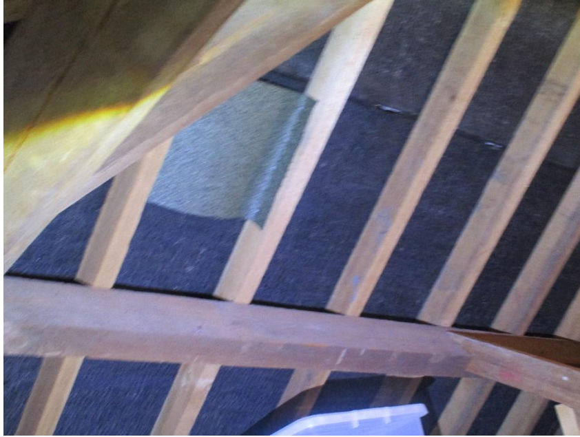
11 Interior – Roof Void – Patch repair to under felting.
