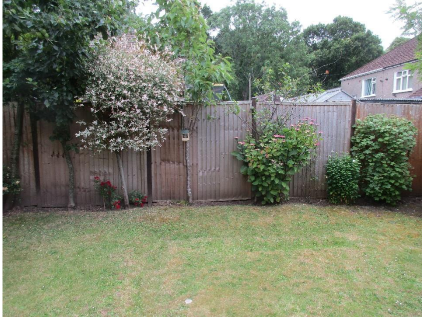
43 Exterior – Rear Boundary.
