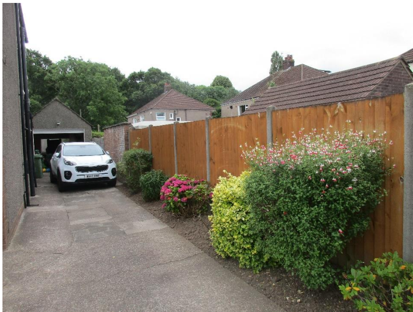
34 Exterior – Front right boundary.
