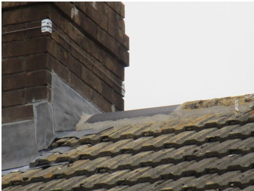
06 Exterior – Replacement ridge tile – fitted to a reasonable standard.
