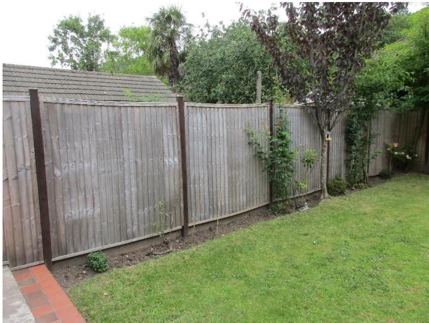
42 Exterior – Rear Left Boundary.
